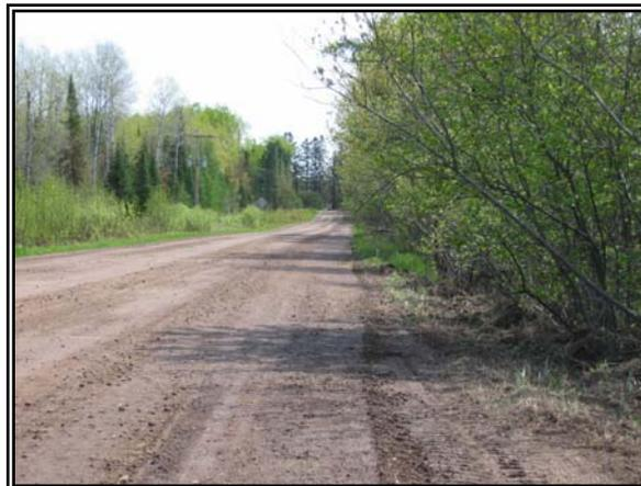
The effectiveness of gravel road grading is dependent on a number of things; including the amount of moisture present in the road base, the current weather conditions and the speed of the traffic using the road.
